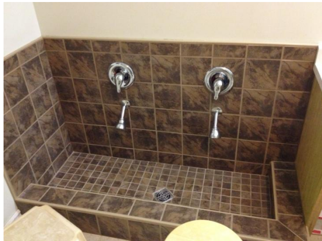
Figure 2 Expanded washroom facility on the main floor.
